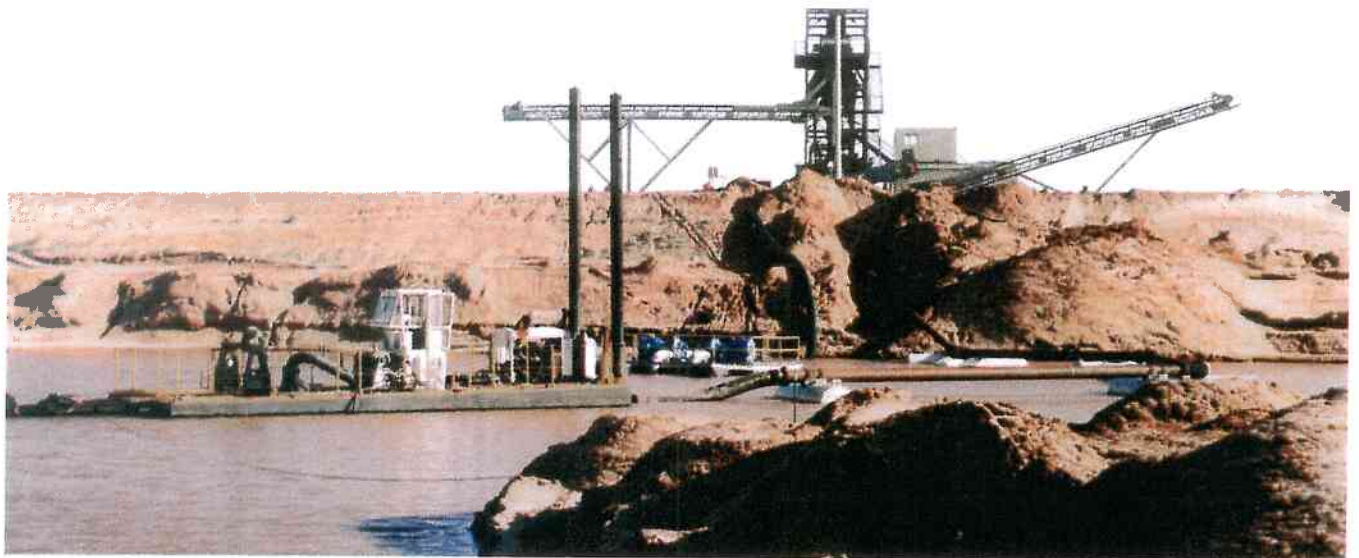
From the Oklahoma side, the mine under construction before production.
